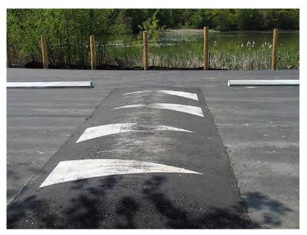
Asphalt speed humps can be installed along Peninsula Road to prevent speeding through the study area. Ideally, these would be placed near crosswalks or intersections to protect pedestrians. These would be a permanent fixture and lost if any upgrades were done to the Peninsula Road.
