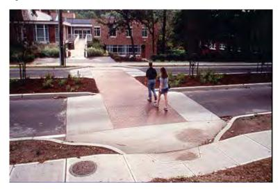
Cars will be required to slow down at a raised crosswalk, allowing pedestrians to cross Peninsula Road in a safe manner. These would be a permanent fixture and lost if any upgrades or resurfacing was done to Peninsula Road.
