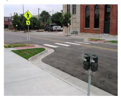
Concrete bulb-outs provide narrower access along the driving lanes, encouraging drivers to slow down. While vehicles may slow down, it also causes conflicts with larger vehicles such as buses, when trying to make a turn around the bulbs.
