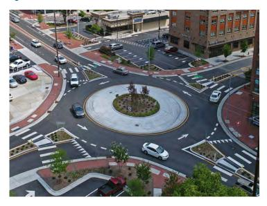
Roundabouts will deter speeding through intersections as vehicles will be forced to slow down to navigate the roundabout. Roundabouts do require a larger footprint to install and may be too large to incorporate into the road ROW on Peninsula Road. Collisions increase at roundabouts as those drivers no familiar with them, may have difficulty navigating through the roundabout.
